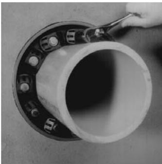
5. Using a hand socket or offset wrench **ONLY**, start at 12 O'Clock. Do not tighten any bolt more than 4 turns at a time. Continue in a clockwise manner until links have been uniformly compressed. (Approx. 2 or 3 rotations)
