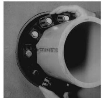
4. Slide belt assembly into annular space. For larger size belts, start inserting Link-Seal modular seal assembly at the 6 O'Clock position and work both sides up toward the 12 O'Clock position in the annular space.
