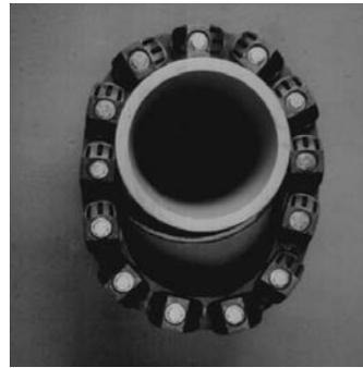
3. Check to be sure all bolt heads are facing the installer. Extra slack or sag is normal. Do not remove links if extra slack exists. **Note:** On smaller diameter pipe, links may need to be stretched.
